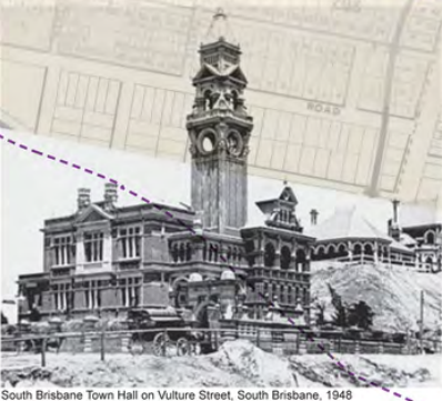
South Brisbane Town Hall on Vulture Street, South Brisbane, 1948
